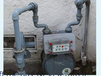
Turn the valve 1/4 turn to shut off the gas. NEVER turn it back on once it has been turned off.
